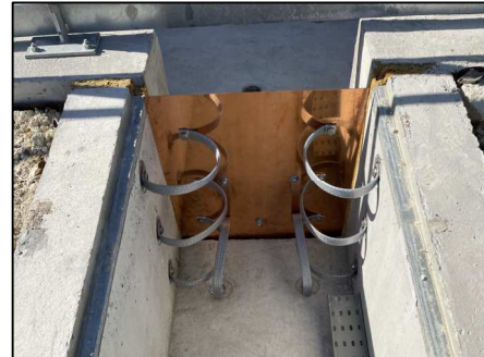
Fig. 4. Copper termination plates.
