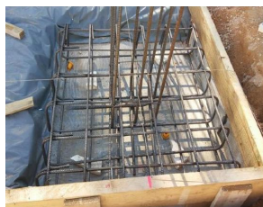
Figure 2: Reinforcement of an isolated footing of the structure.
